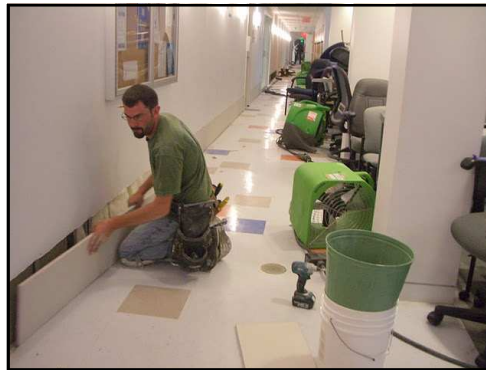
Servpro worker removing a portion of damaged sheet rock in hallway connecting HAB and SUB.
